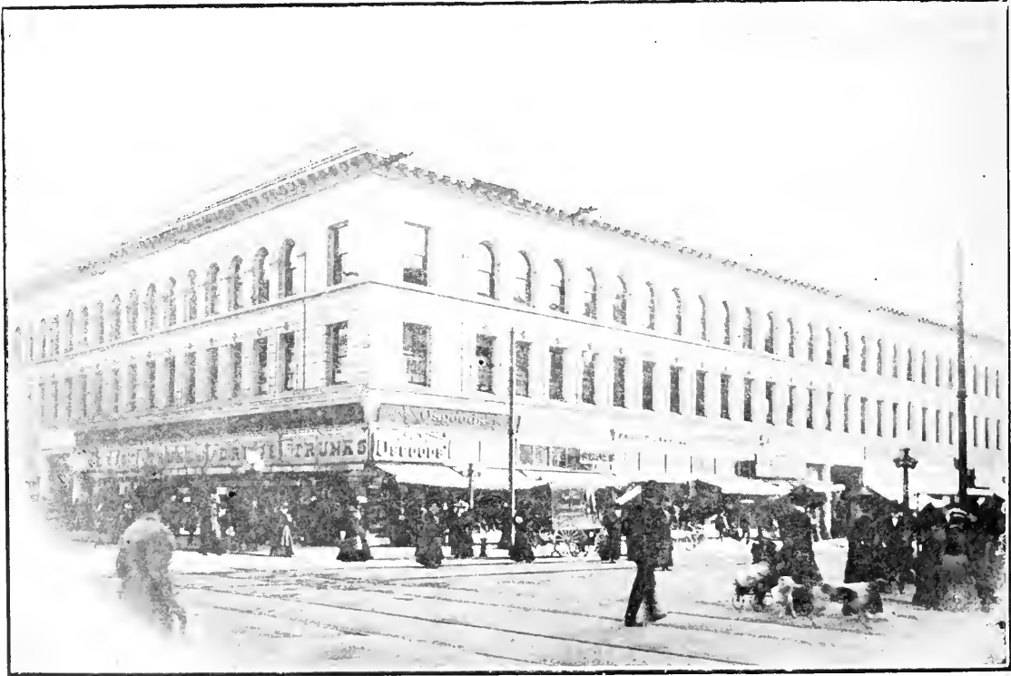
Bacon Building, 12th and Washington Sts., one of the handsome and well-appointed office buildings of Oakland
